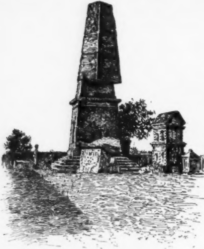
AN EARTHQUAKE STRIKING THE BASE OF A SQUARE COLUMN CAUSES IT TO SWAY CORNERWISE.
